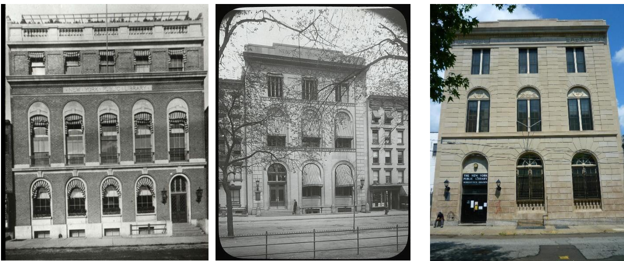
Fig. 2. Carnegie buildings: Hamilton Fish, Tompkins Square, Woodstock
